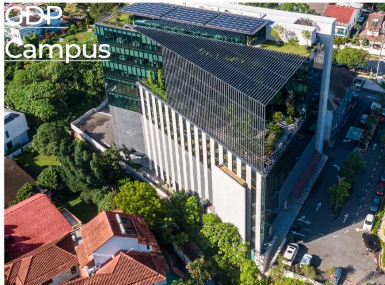
The facade delivers an integrated solution, maximizing daylight, respecting the neighborhood, and embracing passive design with exposed concrete finishes.
