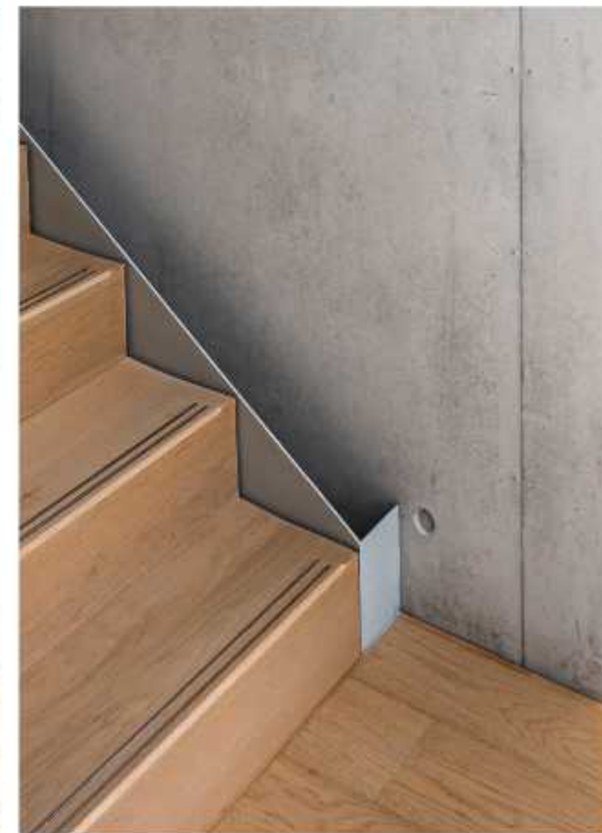
At the base of the staircase, a metal plate marks the transition from the timber stairs to the concrete wall.
