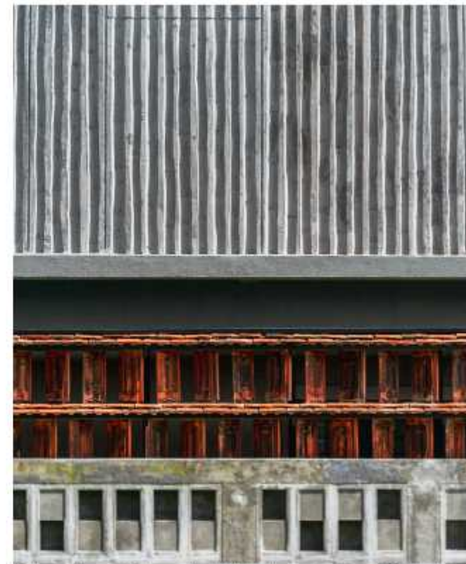
Bamboo lined concrete feature wall made with hard-out bamboo formwork from donated bamboo stems
