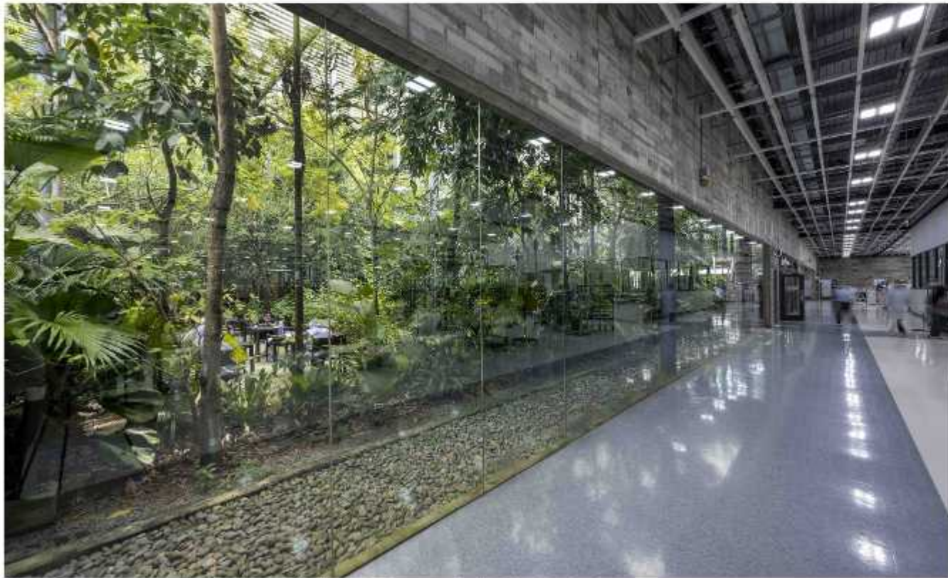
Rainwater is captured on roof gardens, freely falls to pebble-filled catchment sumps, and is directed to storage tanks.
