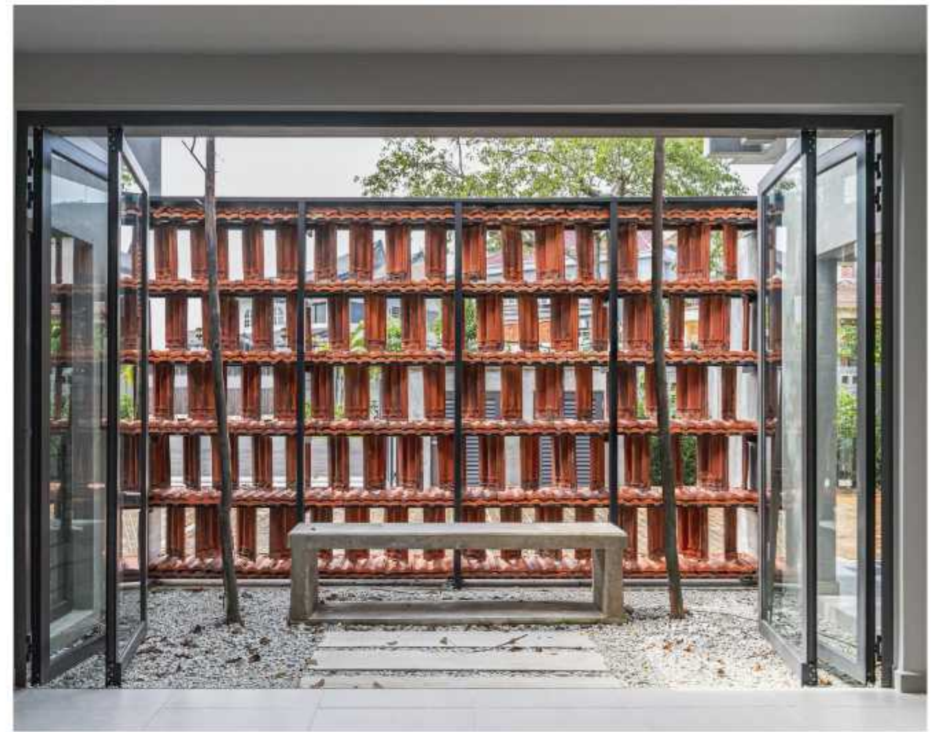
Hand-crafted perforated wall constructed by recycled material
