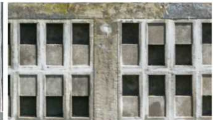
Perforated fence of concrete blocks allow ventilation into courtyard
