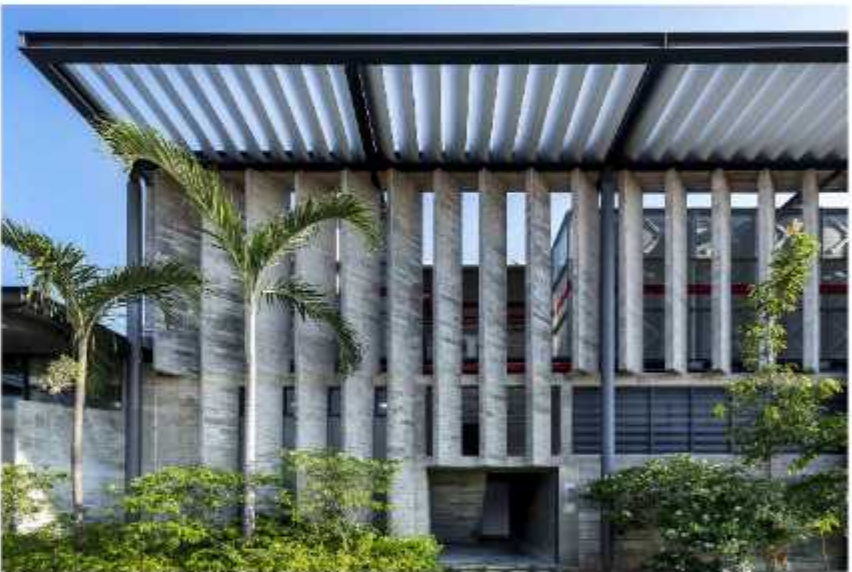
Off-form concrete fins conceal and shade service areas.
