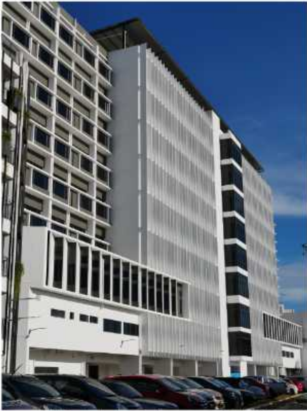
Vertical fins to reduce heat from the morning sun without sacrificing views of the river
