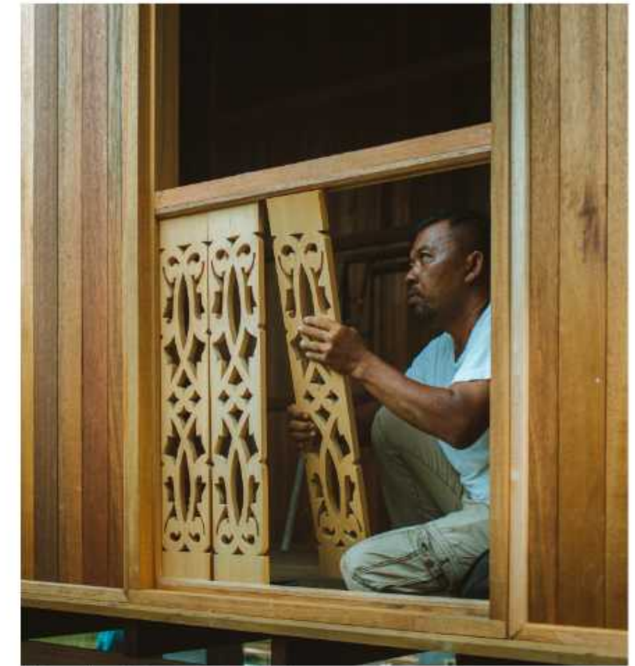
A tukang working on timber house railing in a Malay House
