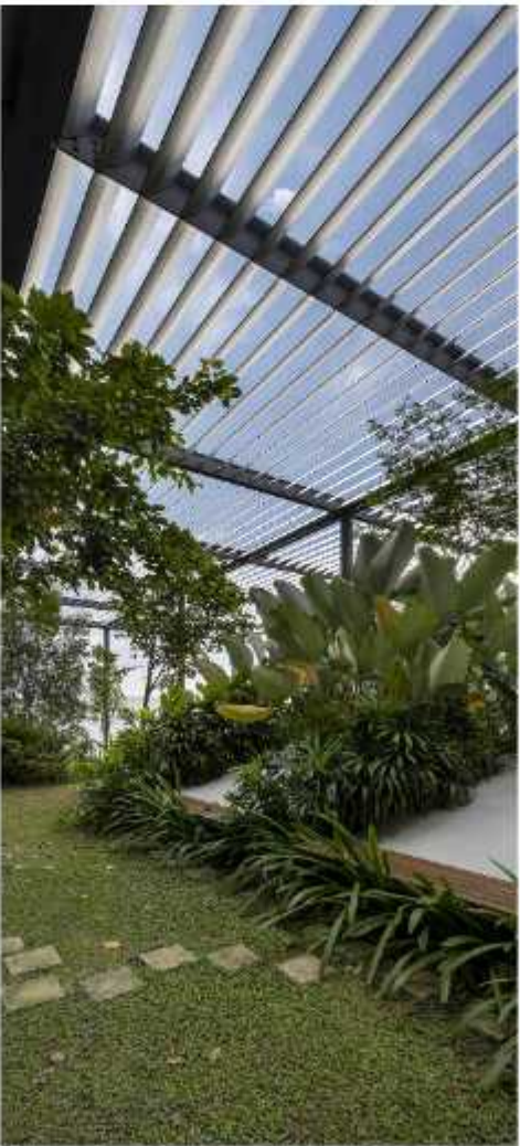
Tight integration of landscape and shading devices mitigates the micro-climate experienced by the enclosure and reduces urban heat-island effect.
