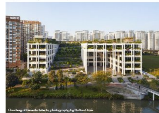
Courtesy of Serie Architects, photography by Hufton Crow Oasis Terraces: a retail, polyclinic and community complex in the Punggol neighbourhood by Serie Architects. (2019)
