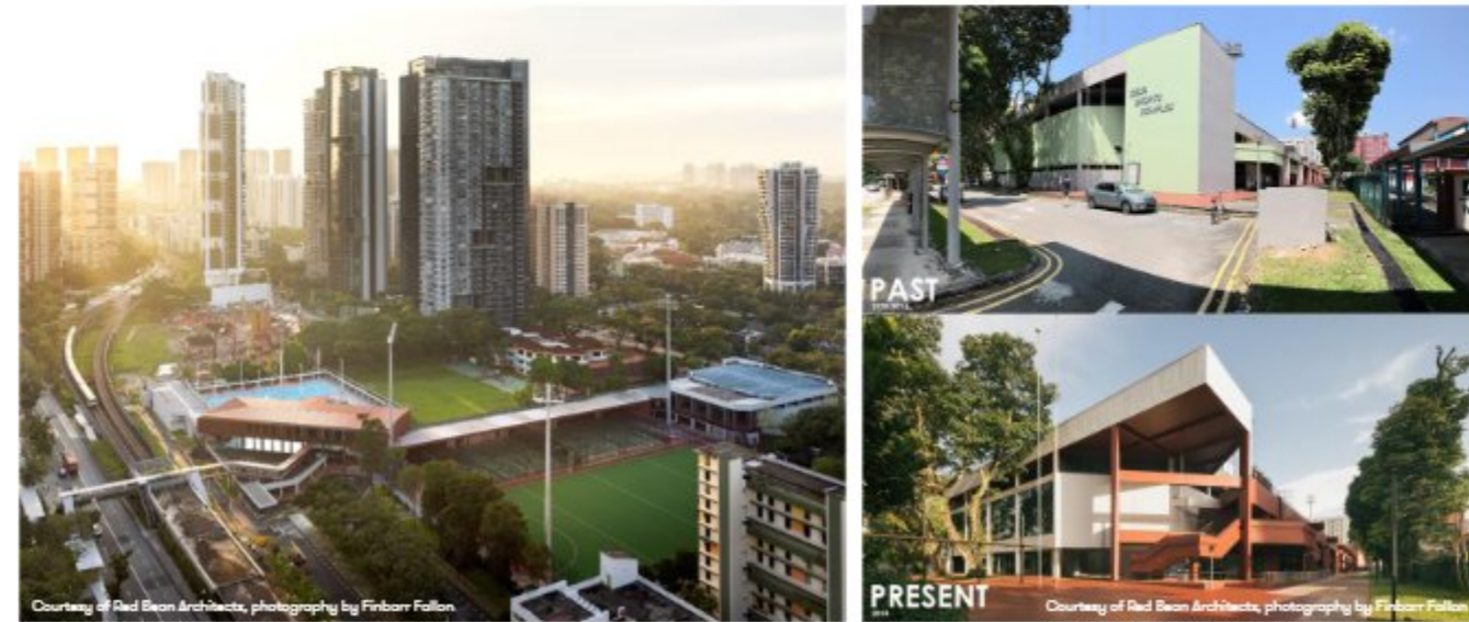
Courtesy of Red Bean Architects, photography by Finbarr Fallon Delta Sports Complex by Red Bean Architects. The project enhances its relevance to the surrounding community through selective stitching, minor demolition and additions to a complex built in 1979.
