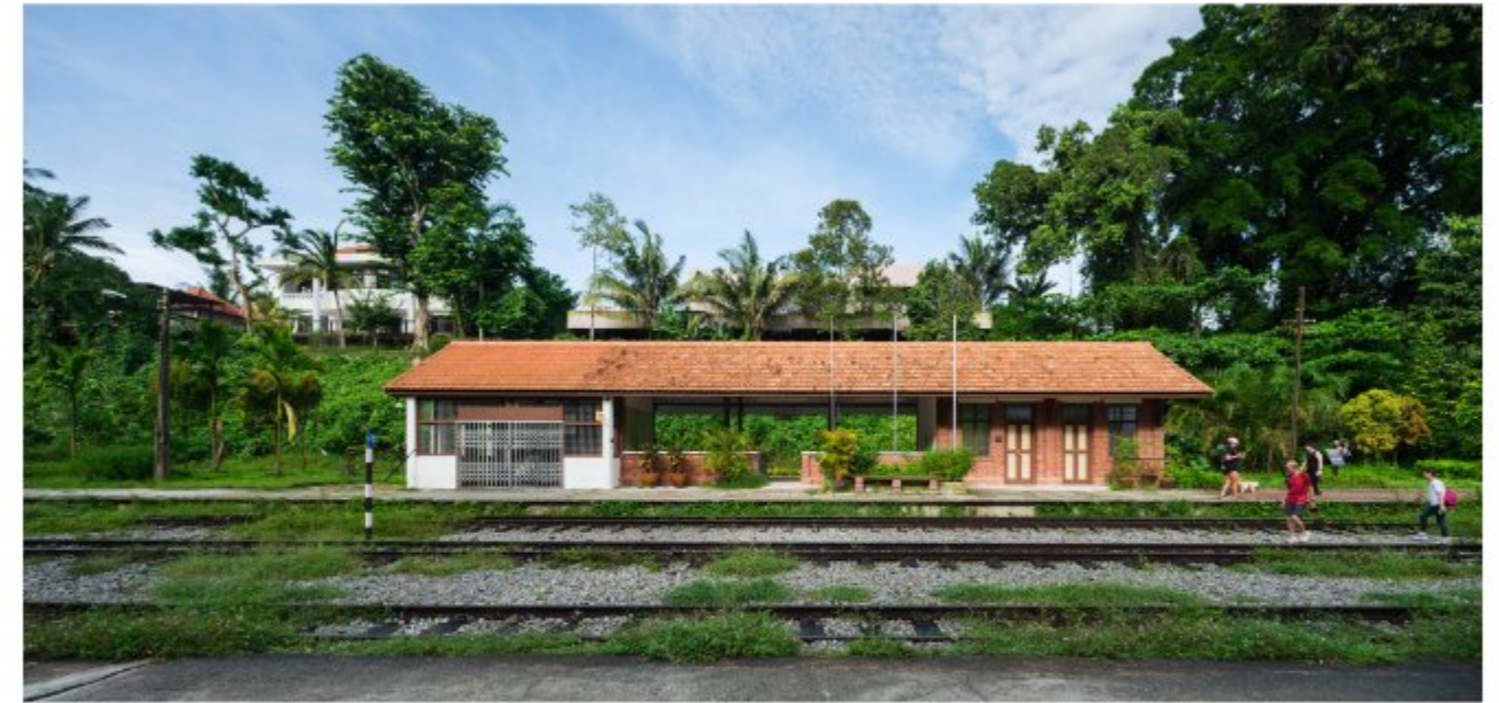
Front elevation of Station house
