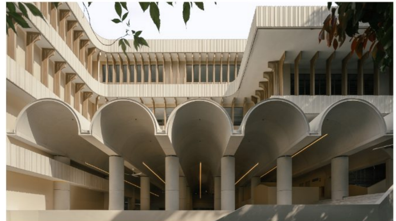
Level 2 Main concourse and new extended barrel vaults
