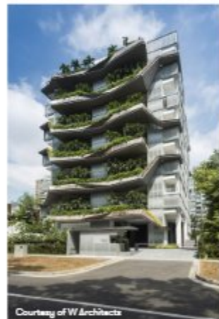
The Oliv by W Architects uses the sky terrace as a front for each duplex unit, reconvening the spatial feel of "villas in the sky"
