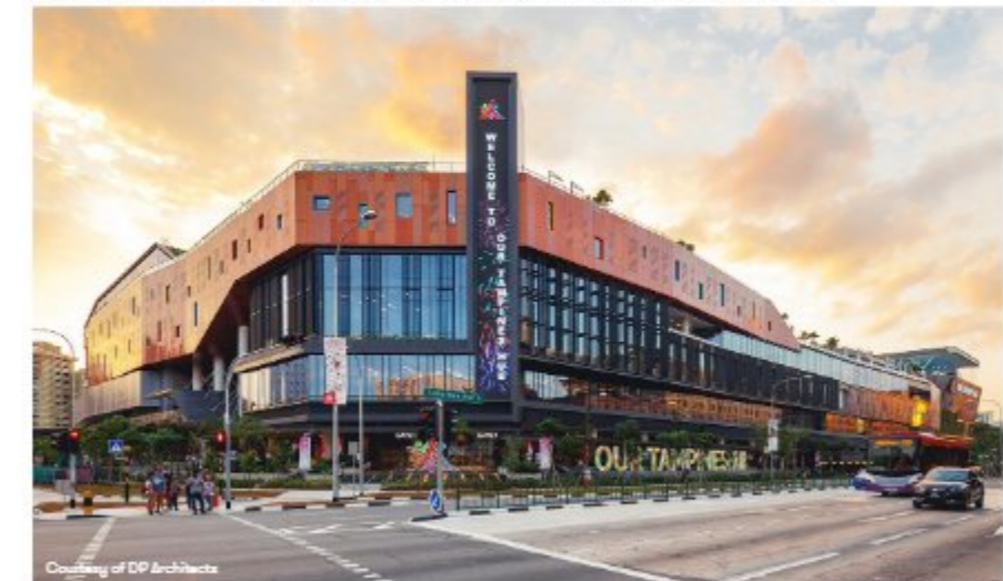
Courtesy of DP Architects Our Tampines Hub, a hub for integrated community, recreational and public services by DP Architects (2017).
