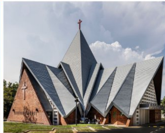
EXTERIOR VIEW: The geometry of the roof's folds dip downwards to wrap the interior with portions touching the ground, reminiscent of anchoring pegs which functionally serve as drainage points for rainwater scaled spaces within and without
