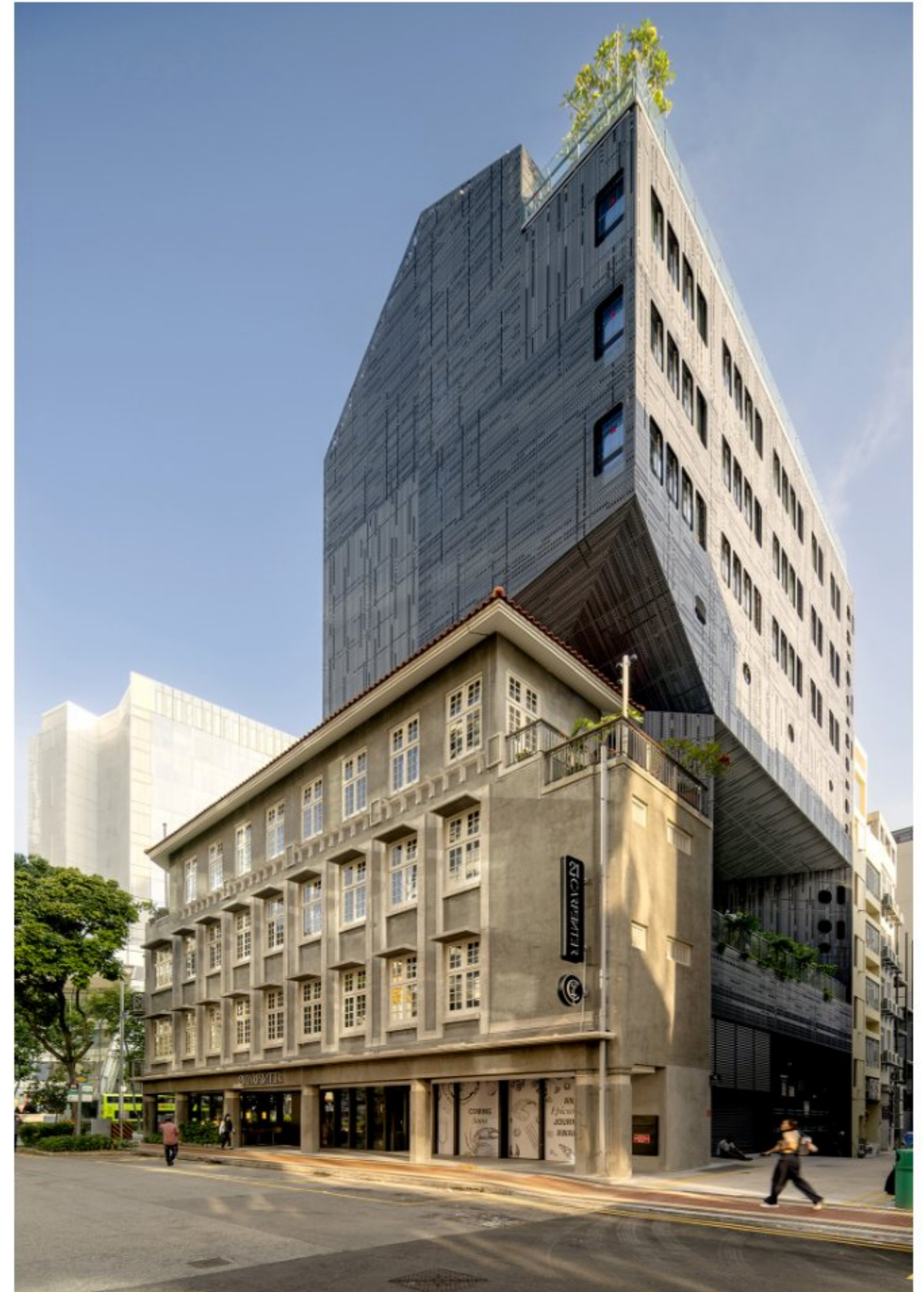
South East corner view showing how the new form arches over and articulates the conserved section
