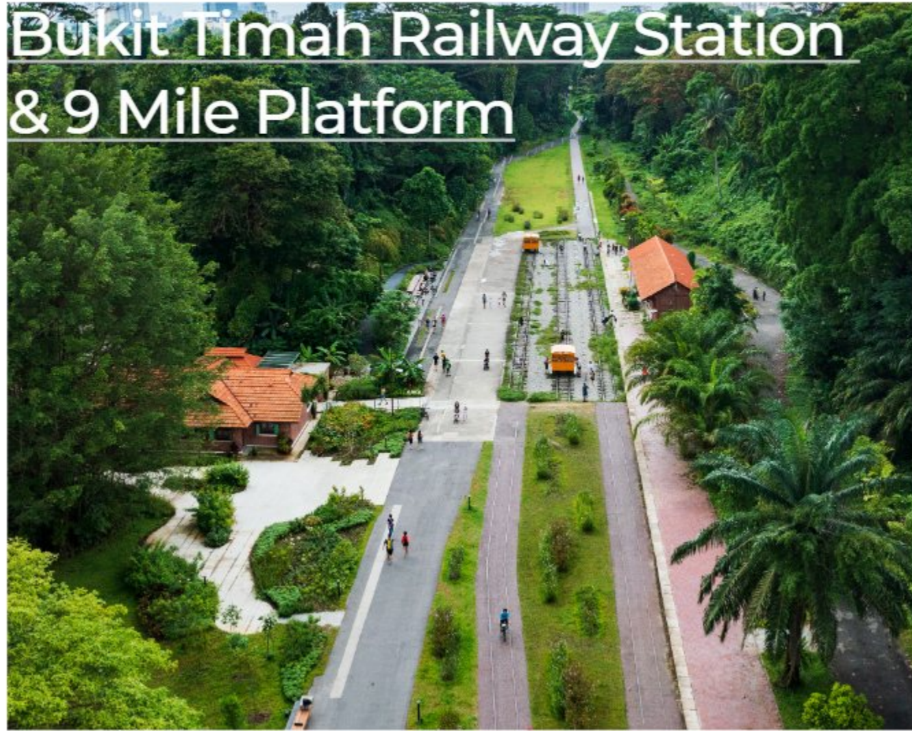
Aerial view of Bukit Timah Station
