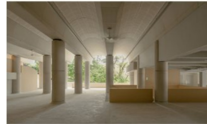
Level 2 Main concourse and barrel vaults
