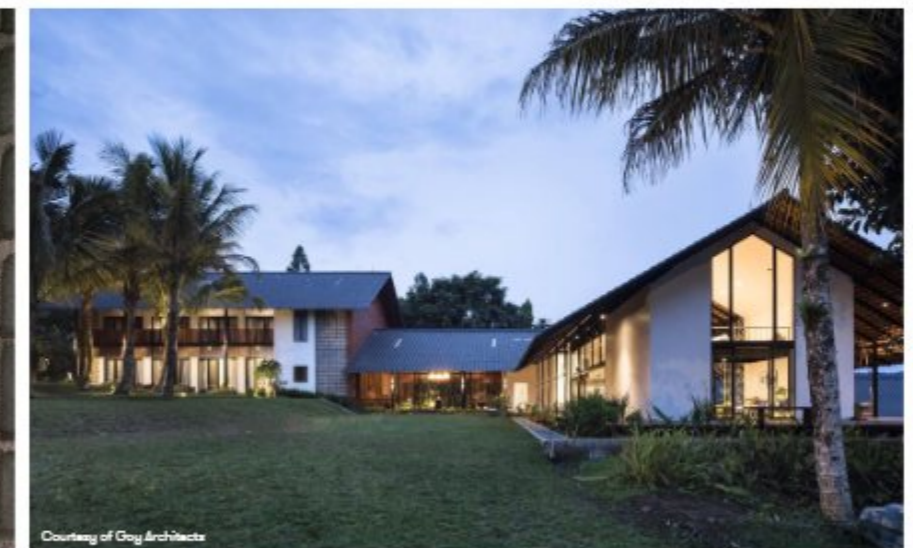
Sukasantai Farmstay by Goy Architects. The building redeploys the simplicity of generous eaves in vernacular regional architecture. It sits gently on its site, using humble materials that reflect indigenous Southeast Asian crafts in a contemporary way.
