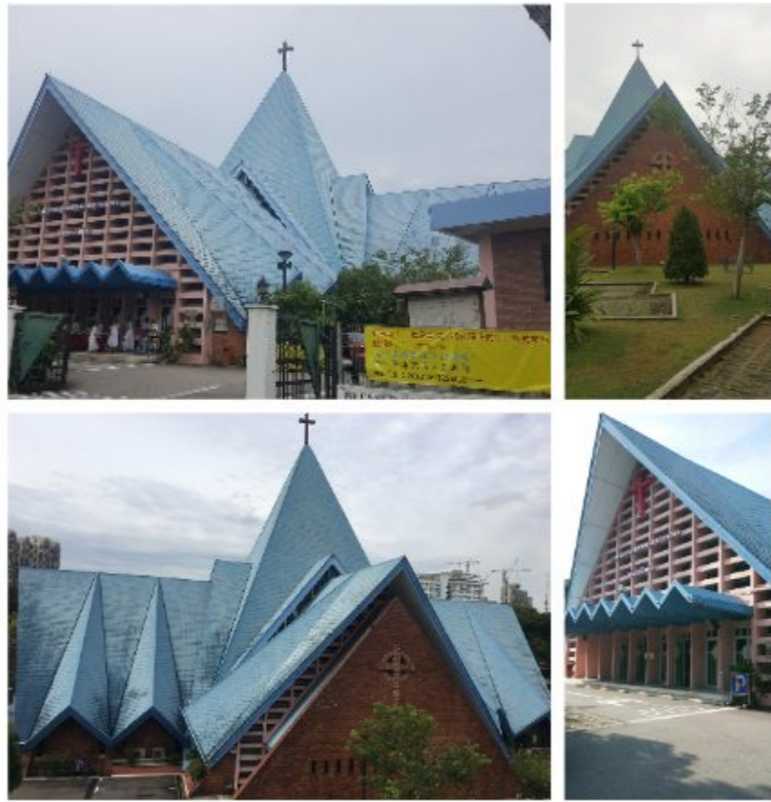
EXTERIOR VIEW: A Modern Aluminum roof replaced the original weathered blue slate tiles to provide a crisp backdrop to the religious artwork.
