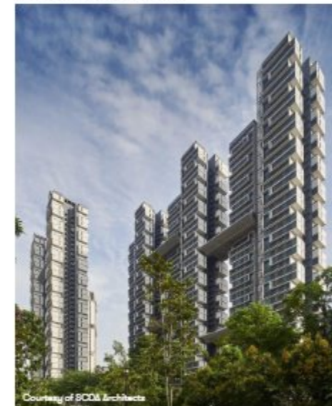
Skyterrace@Dawson by SCDA Architects (c. 2015)
