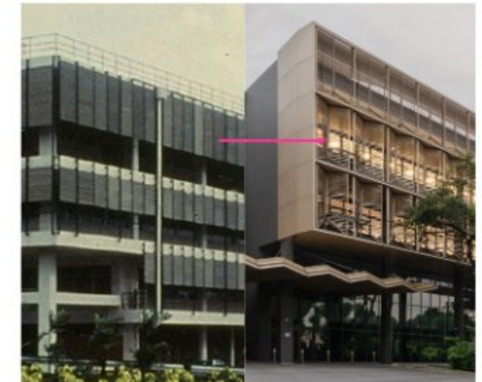
Transposing the old facade elements into the new
