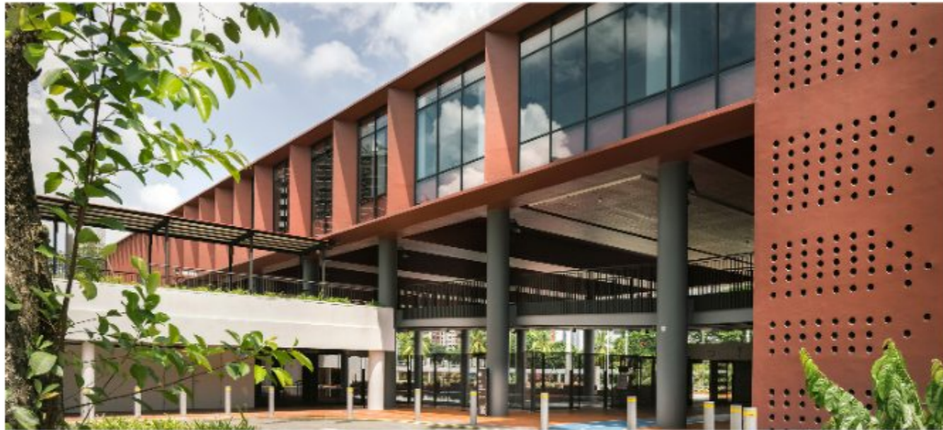
Drop Off Point The main entrance and drop-off is framed by the gym block. Small circular perforations in the concrete staircase wall provide natural ventilation without use of aluminium and glass, 2023. (Finbarr Fallon)
