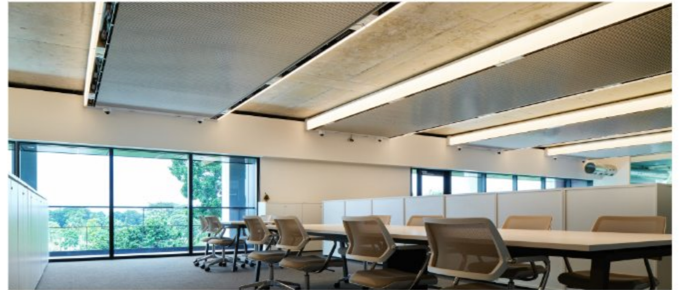
Office interior, with high-performance radiant cooling panels, vertical lighting panels, and glare-free linear downlights.
