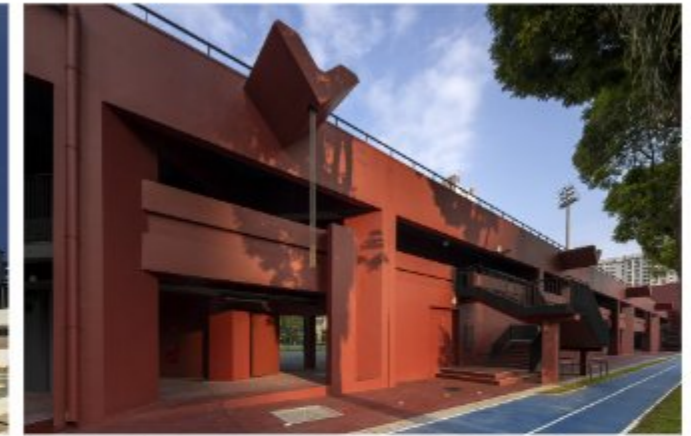
Elevated Promenade The concrete stadium seating has been re-imagined as an elevated promenade that connects the swimming complex to the indoor hall horizontally, with integrated staircases along the pathway providing vertical connectivity, 2023. (Darren Soh)
