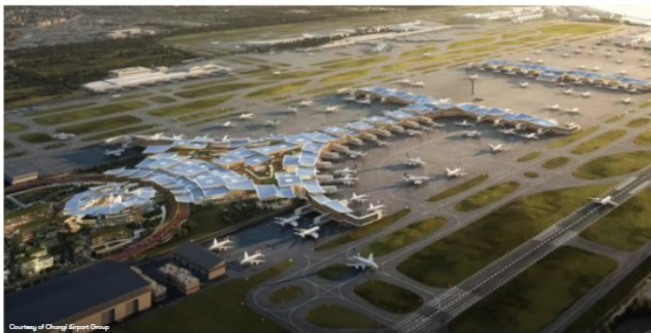
Courtesy of HDB Courtesy of CSYA Studio Courtesy of Changi Airport Group For every major big-ticket investment in Singapore's infrastructure to secure the country's future (e.g. Changi Airport Terminal 5, KPF & Heatherwick Studio), there are equivalent investments in social infrastructure like new housing estates (e.g. Tengah New Town, image below) and markets. (e.g. Jurong West Hawker Centre, by CSYA Studio)
