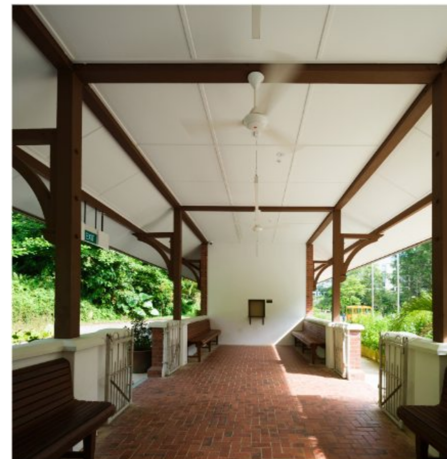
Conserved details of eave corbels and vent ports
