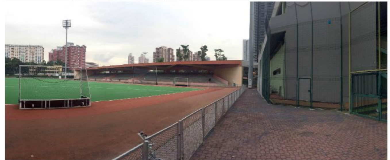
Existing Swimming Pool Complex Existing hockey pitch, flanked by a concrete spectator stand on the left and the rear indoor hall block on the right, with the gym located on the 3rd storey, 2016. (Red Bean Architects)
