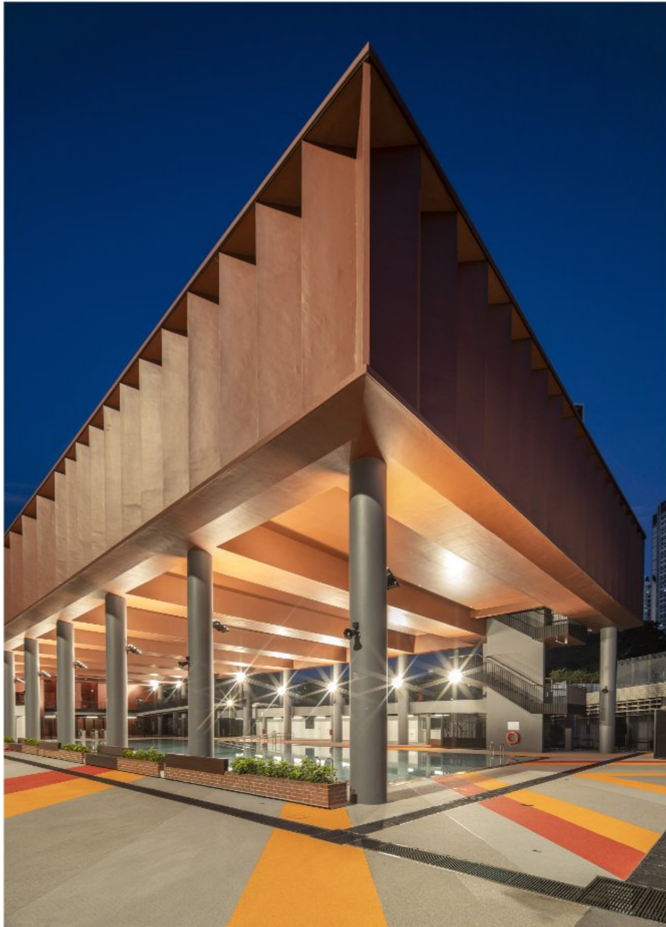
Gym Block Façade The gym block façade integrates sun-shading concrete fins against the east and west sun with glazing always facing north and south. The solitary fin touching the corner is a result of this logic, 2023. (Darren Soh)
