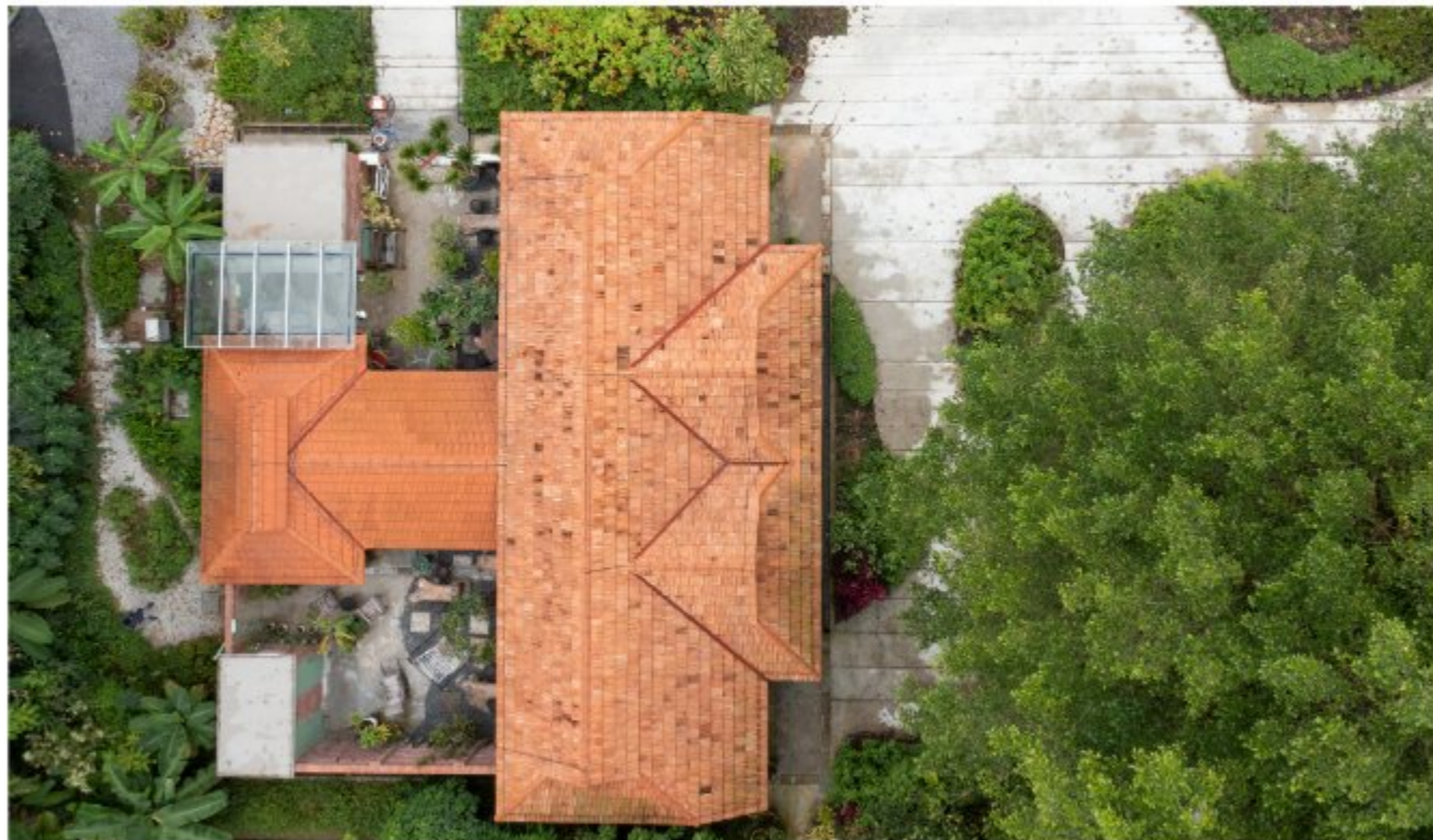
General view of Station Ticket Office
