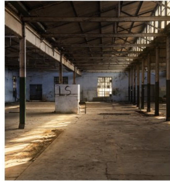
View of the Industrial structure before intervention
