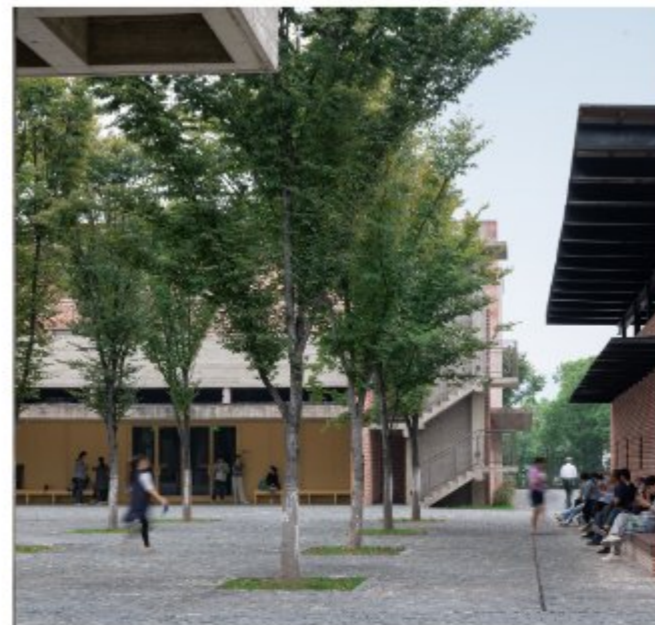
Eaves and seats around zelkova tree square
