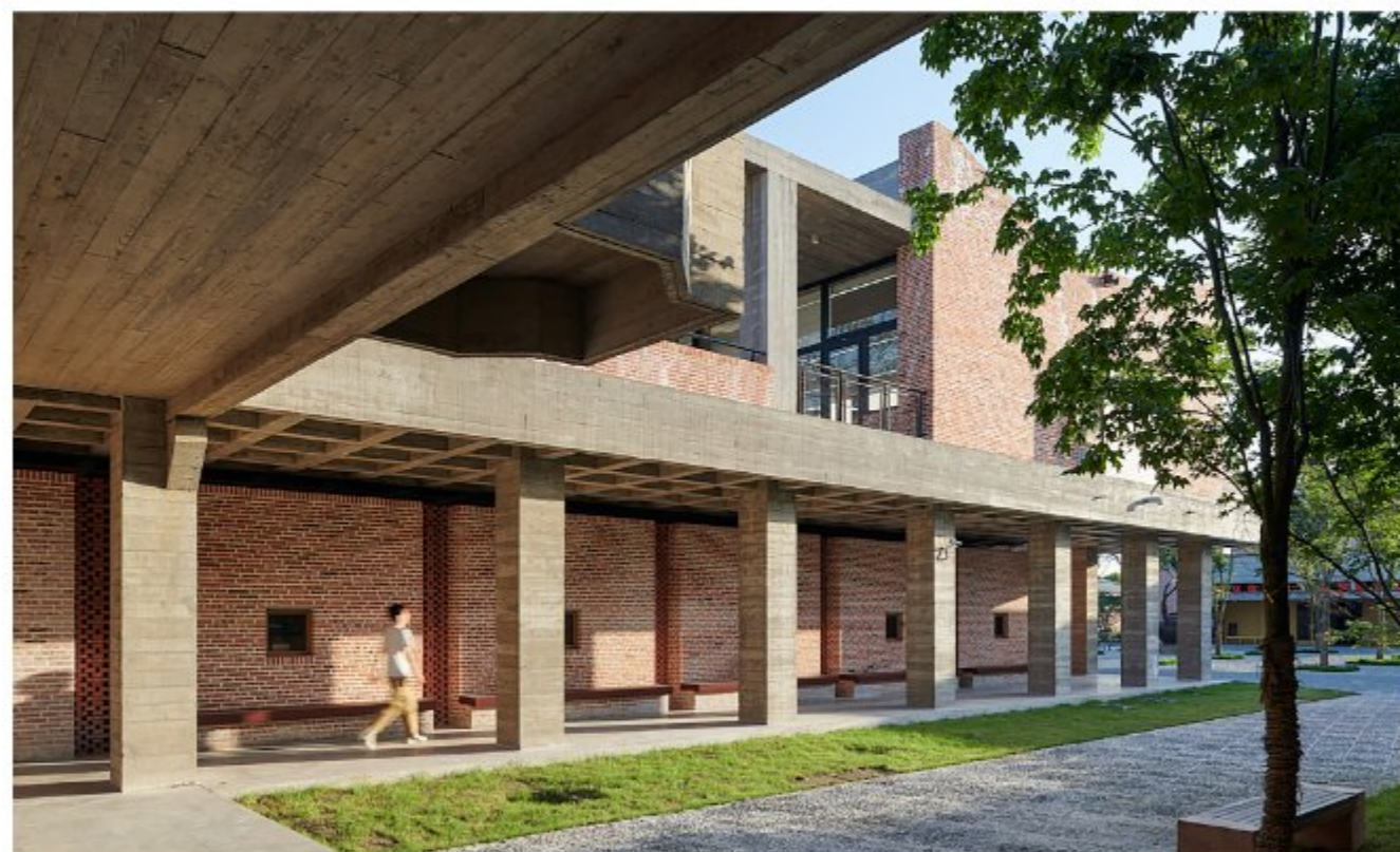
The side porch along the exhibition building towards the central Zelkova tree square
