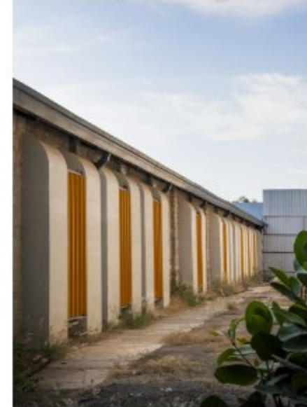
Exterior view of a restored industrial shed
