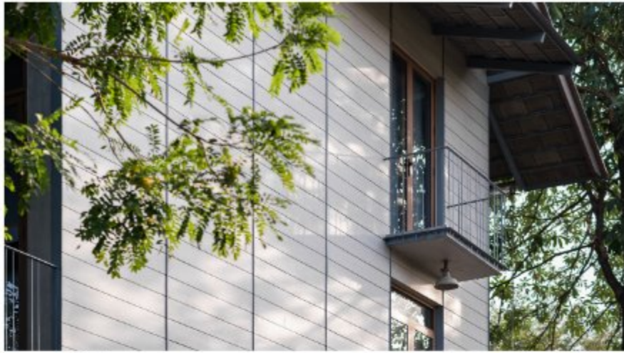
Front Facade Detail
