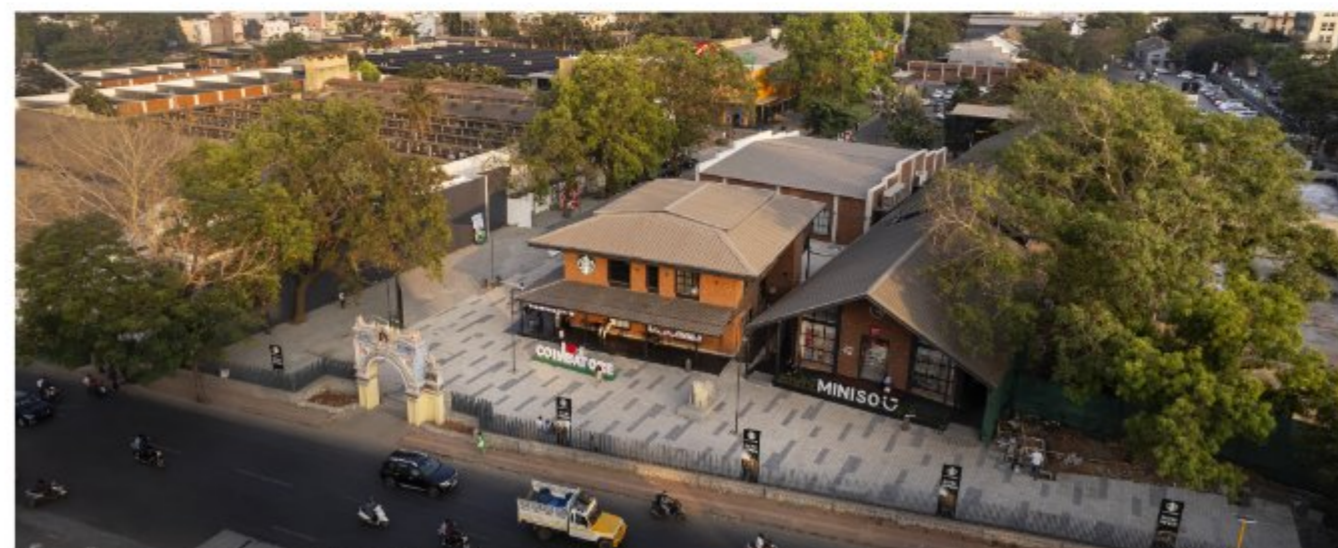
Birds-eye view of the pedestrian entry to the Lakshmi Mills redevelopment premise.
