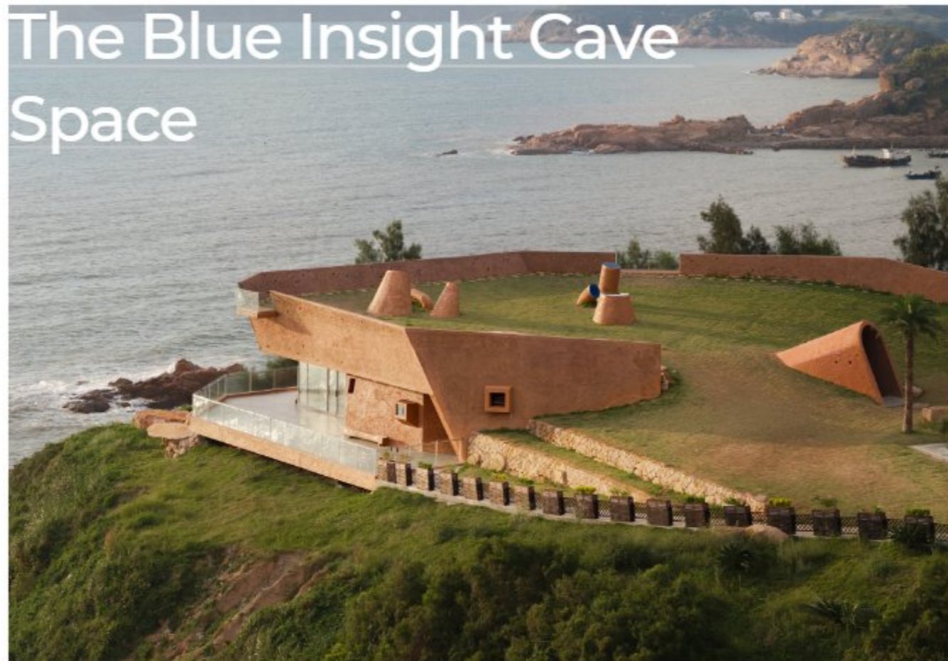
The building adopts a soil covering form, and the main part is semi-underground
